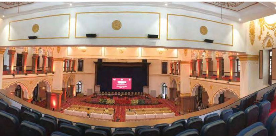
Minto Hall auditorium's system consists of Left-Right asymmetrical RoomMatch arrays, with the left array comprising RM602810, RM602820, and RM602840 modules, while the right array comprises RM286010, RM286020, and RM286040 modules
