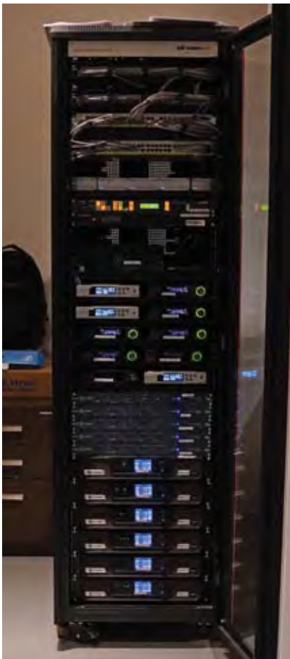
Racks placed with integrated modules for control, video conferencing, lightning, network, signal management and displays
