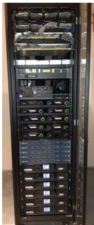
Racks with integrated modules for control, video conferencing, lightning, network, signal management and displays
