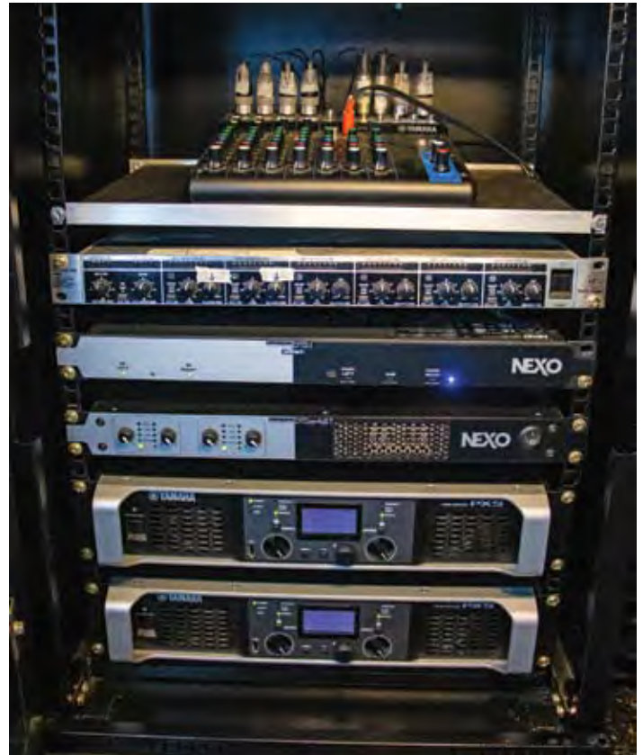
The loudspeakers used in the main area are powered by Nexo DTDAMP and PX5 Amplifiers
