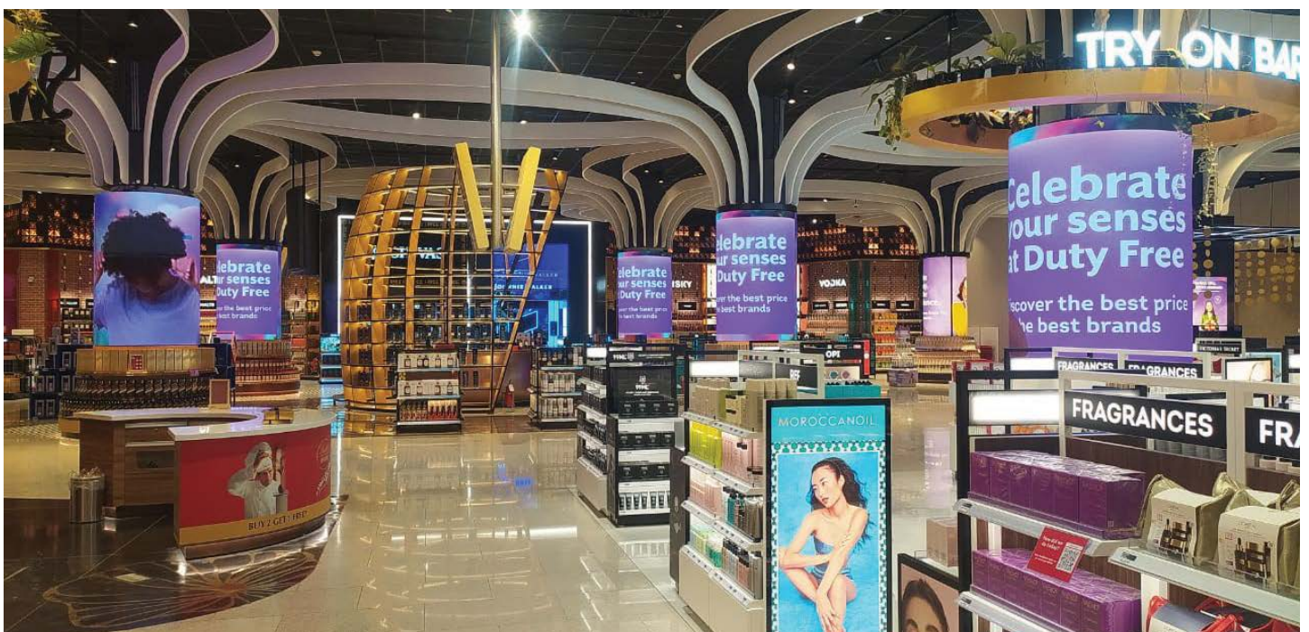
Xtreme Media installs Flex and Nyx Series of 2.5mm and 3.9mm pixel pitch – 13 LED displays at International Airport, Bangalore
